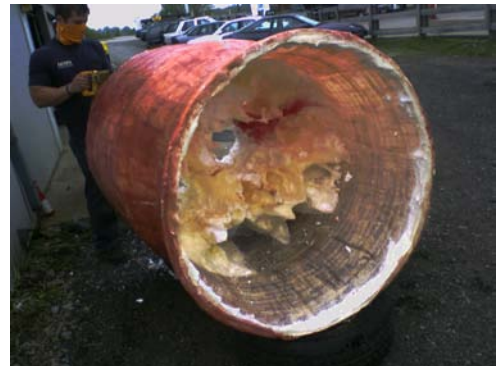
Figure 2.2: Removal of Styrofoam from tower shell
